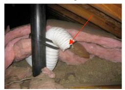
The bathroom exhaust fan that terminates in the attic space (see photo left) should be vented to the exterior of the building to help reduce moisture levels in the attic space.
