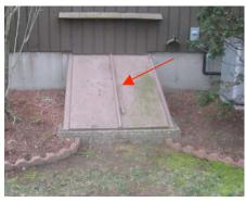
We also recommend that you seal the vulnerable areas of the bulkhead entrance (see photo left) and cover it in the winter, as required to help ensure a weather tight seal.
