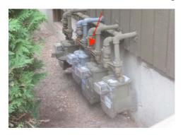
The main fuel (natural gas) meter and shut off valve are located at the front of the exterior of the building, between units 83-A and 83-B. (see photo left-arrow indicates shut-off valve)
