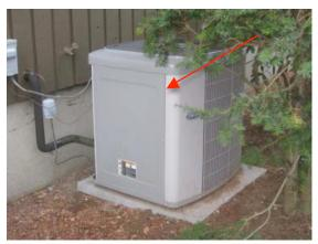
Carrier brand, electric, conditioning system compressor (serial # 0303E07578- see photo left) was not activated due to the low exterior temperatures. Most manufacturers recommend, in order to avoid damage, that these units not be activated when exterior temperatures fall below 65 degrees Fahrenheit. Obtain some type of guarantee from the seller that this unit will be in good working condition when needed. For maximum efficiency, service
