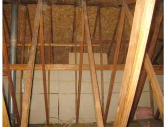
The attic framing and roof structure consists of 2" x 4" roof trusses installed 24" on center and 2" x 4" floor boards installed 24" on center. The roof has been sheathed with oriented strand boards ("OSB") - see photo above.
