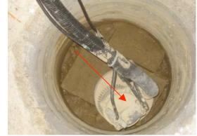
install a battery operated back-up system for the sump pump to help ensure its operation during a power outage.
