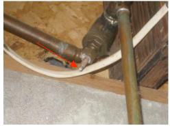
The missing, valve handle for the main water shut off valve should be replaced for your safety and for your convenience.
