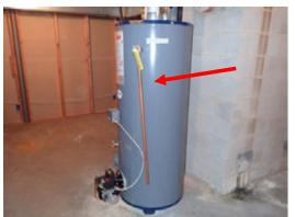
The water is heated by an independent, 70-gallon, oil-fired, Bock brand, water heater (serial # 03083180T/model # 71E - see photo left) with a recovery rate of approximately 185 gallons per hour. The hot water supply system was evaluated and found to provide adequate amounts of hot water to all fixtures tested, at the time of this inspection.
