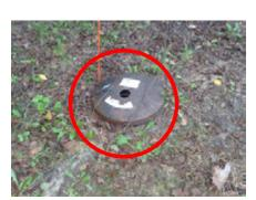
A propane gas (LPG) tank was buried at the rear left planting area of the house (see photo left). The shut off valve is located under the top cover of the buried tank (see photo right).
