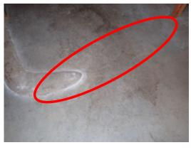
preventing evaluation of the oil supply pipes. If the oil lines are not protected with plastic sheathing, the copper pipes are likely to be adversely affected by their contact with the concrete. It should be noted that oil could leak from these pipes below the concrete. We recommend that you have your oil supplier re-route the oil lines as required to remedy this condition and that the pipes be encased in protective sleeves to help prevent damage to the pipes.
