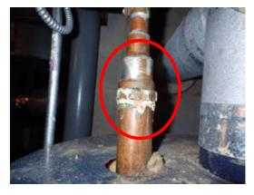
Corroded fittings were observed at the top of the water heater. When the water heater is serviced, make any necessary repairs to help prevent leaking and consequential damage.
