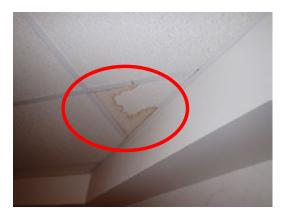
stains watermarks were observed on the ceiling in the finished basement exercise room (see photo left for one example area) the and on chimney structure in the rear right unfinished
