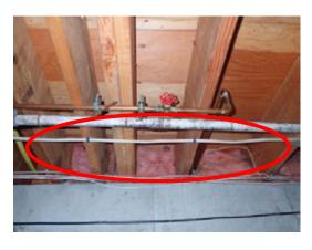
Black, microbial growth-type staining observed in the basement on the PVC water supply pipes servicing the sprinkler system (see photos right and left for This examples).
