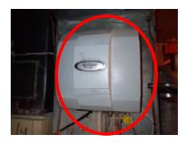
The humidifiers installed on both furnaces (see photos left and right) should be serviced in accordance with the manufacturer's recommended procedures. The humidifiers' bypasses should be open during the heating season and closed during the cooling season.
