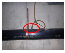
can enter the air handler and possibly be distributed into the living spaces. We recommend rerouting the drains to the exterior of the house and sealing the waste pipes to prevent the gases from entering the basement space.
