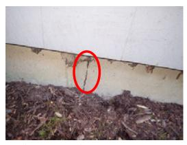
The foundation walls are poured concrete and concrete blocks. Settlement cracks were noted in the foundation at the time of the inspection (see photos left and for right examples).
