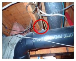
The condensation drains for the air handlers/evaporator units in the basement drain into the waste piping (see photos left and right). This is not recommended because when the "drain traps" dry out during the heating season, septic gases
