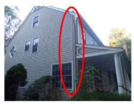
This house has been fitted with a radon mitigation system (see photo left of exterior components and see photo right of manometer the and piping inside the house). The system did not appear be to
