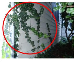
structure and to the siding as well as the foundation and to the vulnerable exterior cladding and the materials beneath the siding and trim components in these areas. The foliage can also provide an inviting environment for moisture and insects. Consider removing the offending vines.
