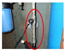
condition is usually the manifestation of a space that requires additional ventilation and/or dehumidification. Add ventilation and/or dehumidification as necessary to help prevent microbial growth.
