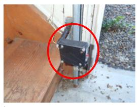
We recommend that you lower the "photo-sensitive eyes" servicing the right-most garage door (see photos left and right) to 6" above the garage floor to help allow them to function as designed and to
