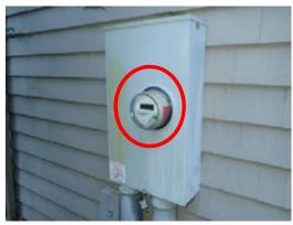
400-ampere (2 x 200 amperes), 120/240-volt electrical system enters the building via underground cables. The electric meter is located on the the exterior of
