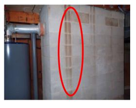
basement area (see photo right). Inquire with the owner as to the cause for the staining, when it occurred and what measures were taken to help ensure that the staining will not recur.
