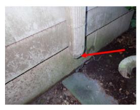
All rain leaders terminating into in-ground receptacles must remain free flowing all at times (see photo right for example of an in-ground receptacle). Underground systems are
