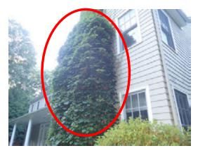
The tendrils of the vines clinging to the rear left center chimney and to the siding as well as the foundation (see photos left and right for examples) can damage the chimney
