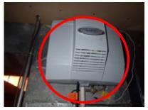
Humidifiers are prone to leaking (there was evidence of past leaking under these two humidifiers on the ductwork and on the furnaces' jackets that appeared to be from previously installed malfunctioning humidifiers). If leaking recurs, the humidifiers should be serviced promptly to prevent damage to the heat exchangers and/or to the ductwork. We do not recommend the use of this type of humidifiers.
