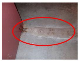
The oil supply pipes supplying the two furnaces (and the water heater) are with covered concrete and they under the run concrete slab floor photos left (see right for and example areas),
