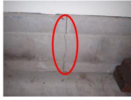
Settlement cracks are not uncommon and are usually the result of improper soil grading around foundations. This condition is presently not a structural problem. It must be noted that settlement cracks could develop into structural cracks. Periodic inspection of these cracks and proper care should prevent future problems. These cracks should be filled from the exterior with a suitable material to help prevent seepage and they should be monitored for any further movement.
