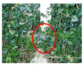
vulnerable to clogging and should be checked annually. The rain leaders that do not terminate into an in-ground receptacle (see photo above left for example) need to be extended as far away from the foundation as practical to prevent roof water from collecting against the house and seeping into the lower level.
