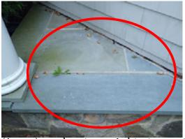
We observed gaps, voids and open mortar joints as well as a loose slate stone in the front right corner slate stone surface (see photo left) that should be repaired to help prevent water infiltration and damage to the patio and potentially to the patio substrate, at-grade and sub-grade foundation and interior spaces.
