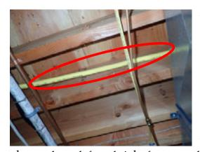
OmegaFlex brand, "Tracpipe" corrugated stainless steel tubing (CSST) was observed in basement, apparently servicing the propane-fired kitchen cook top burners (see
